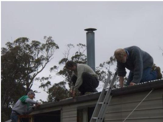
Hopefully this will stop the leak. The guttering was unclipped and cleaned, and a downpipe fitted at the rear to take excess water away from the shack.
