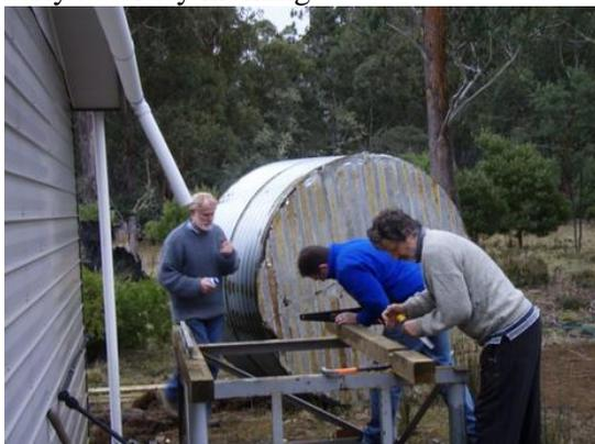
A talented band of carpenters rebuilt the deck with treated timber and leveled it after discovering that the steel base was sloping distinctly towards Bothwell. An overflow was
